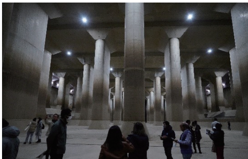
In the Metropolitan Area Outer Underground Discharge Channel 首都圏外郭放水路内にて
