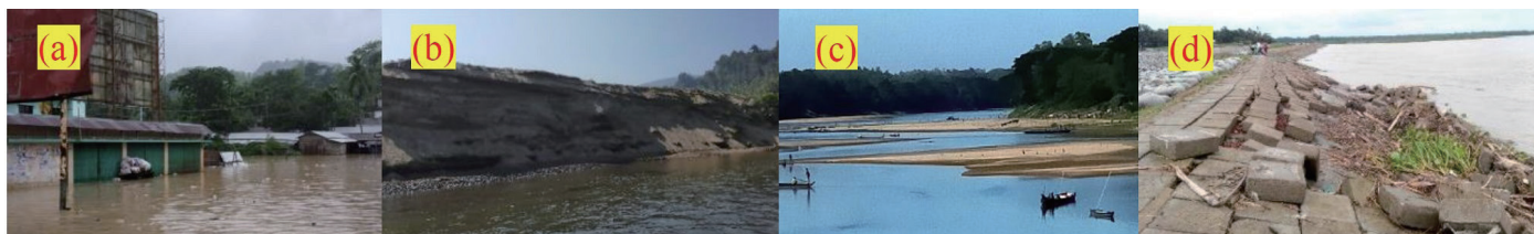
Figure 2 Problems in Sangu river (a) Flood in 2015, (b) Bank erosion, (c) Sand bar, and (d) Damaged river bank protection works
