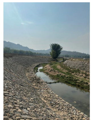
Figure 1 Nikas kholo protection work, Surkhet
