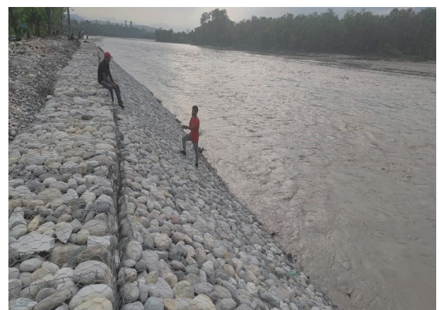
Figure 2 Bheri River Training Work, Surkhet
