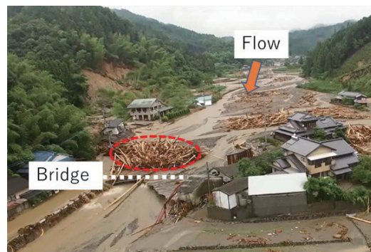
Photo 2 A section of the Akatani River damaged during the 2017 torrential rain disaster in northern Kyushu. The photo was taken by the Geospatial Information Authority of Japan.
