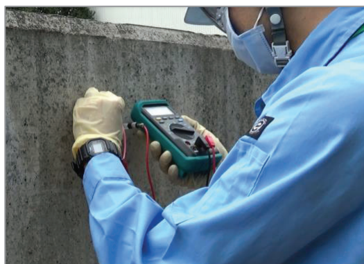
Photograph 2: Measurement using a chloride sensor
