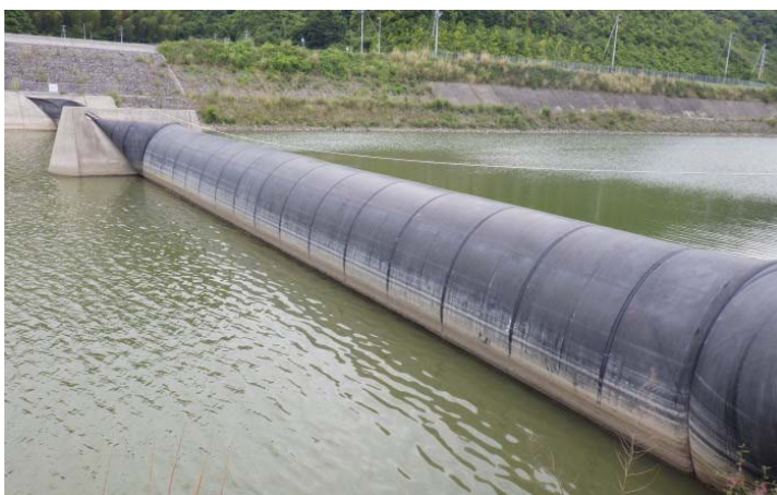
Figure 6: Overview of inflatable rubber gate (rubber dam)
