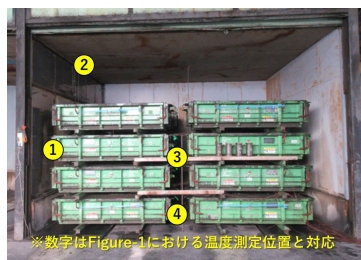
Photograph-3 Example of steam curing facility
