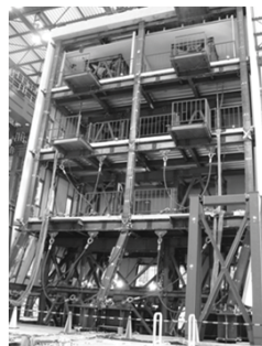
E-Defense Steel Collapse
