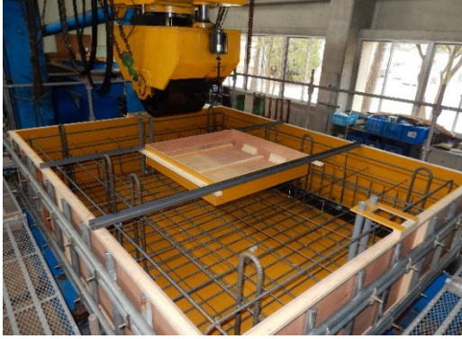
(a)母材の型枠と配筋
