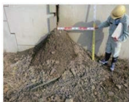
Example of outflow of reinforced-back-surface soil (a simple maintenance method is required)
