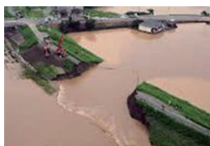
Levee breach by piping
