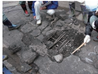
Deterioration of the road bridge deck due to frost damage
