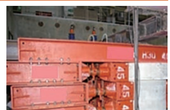
Emergency restoration technology for shear fractures of the bridge seats (emergency restoration method using H-section steel that is easily available)
