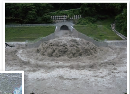
Sediment bypass tunnel (Outlet of Miwa Dam facility)
