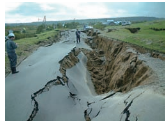
Collapse of embankment on the peat ground due to liquefaction
