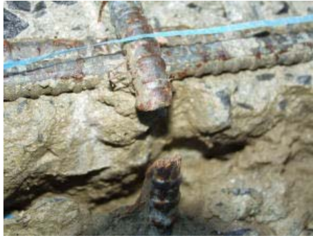
Figure 1: Fractured stirrup
