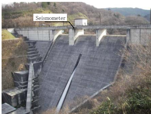
Photo. 1 Downstream face of Hakkagawa Dam
