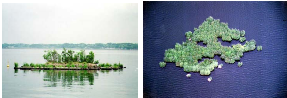
Figure 2. Dry-concrete AFI in Lake Kasumigaura (left) (photo: Maeda Environmental Art), Wet-without-frame AFI with coconut fiber plant base (right) (Komoro regulating pond)
