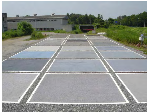
Figure 5: The 4 m x 4 m pavement specimens
