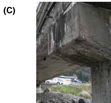
Anatomic survey for an overpass that suffered from salt attack.
