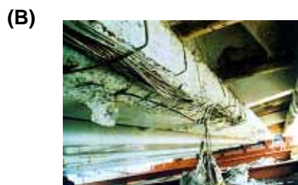
Anatomic survey for an overpass that suffered from salt attack.
