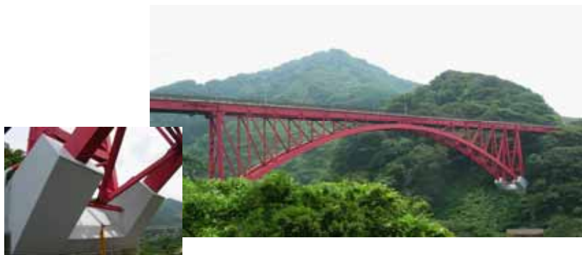
Figure 13 A long span bridge did not undergo damage during the 2007 Niigata-ken Chuestu-oki earthquake (Mj6.8) because of seismic reinforcement supported by the PWRI.
