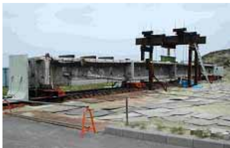
Figure 8 Field load test of a damaged member from an older bridge
