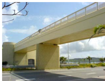
Figure 1: View of the Okinawa Road Park Bridge
