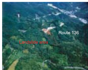
Fig.1 Landslide view from the sky (Photo by Shizuoka prefectural government; August 7, 2007)
