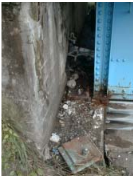
Photo 5 Effectiveness of PC Cable Type Unseating Prevention Devices
