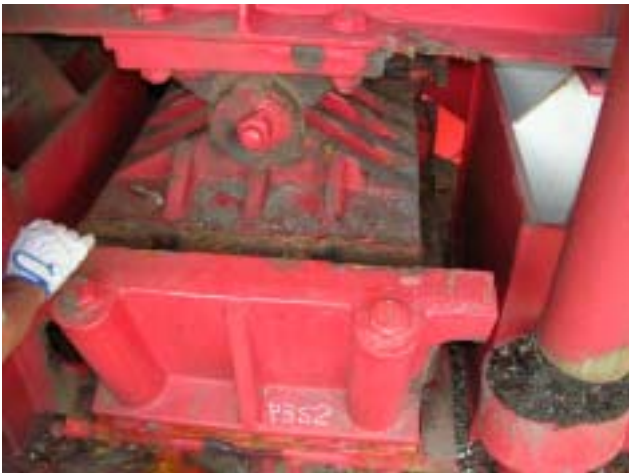
Photo 12 Deformation of Shear Keys and Pin Caps of Bearings
