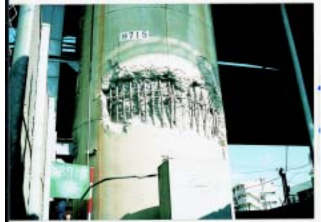
Photo 2 Pier P715 of Hanshin Expressway [6]
