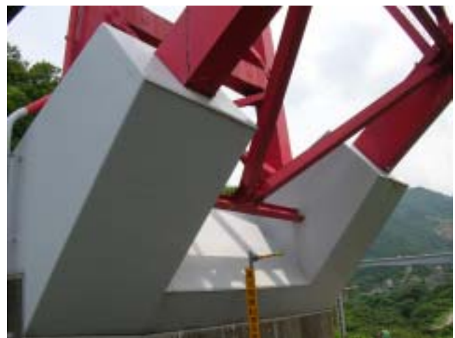
Photo 10 Retrofitted Springing Section of Arch Rib (Concrete Jacketing)
