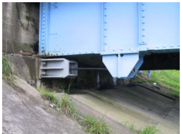
Photo 5 Effectiveness of PC Cable Type Unseating Prevention Devices
