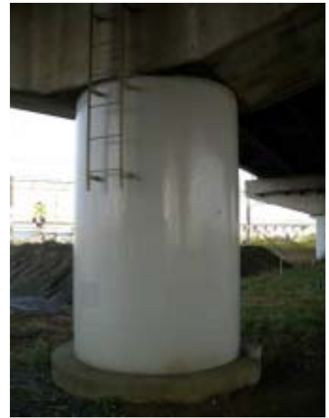
Photo 7 Retrofitted Columns with Steel Jacketing (No damage)
