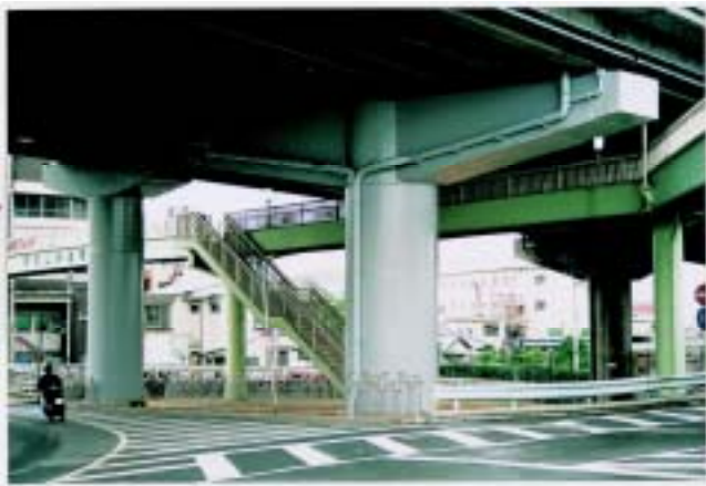
Photo 1 Retrofitted Pier P714 of Hanshin Expressway [6]
