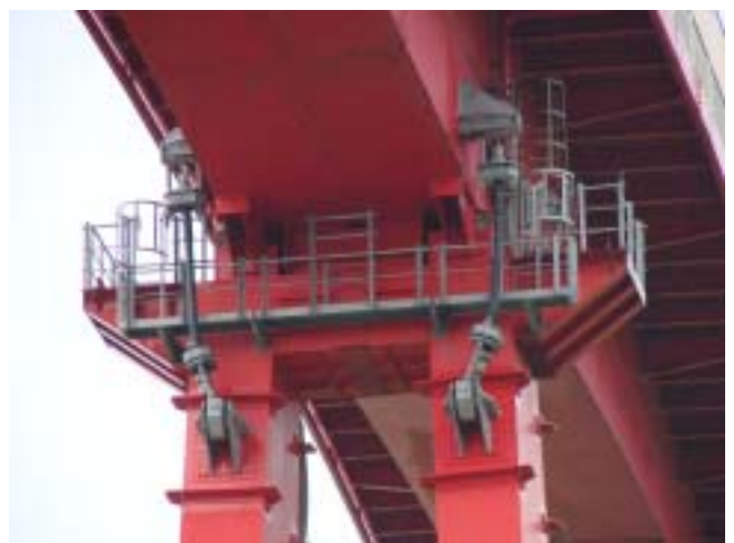
Photo 13 Unseating Prevention Devices (Cable Restrainers in Longitudinal and Uplift Directions)
