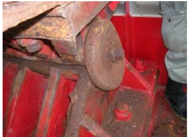
Photo 12 Deformation of Shear Keys and Pin Caps of Bearings
