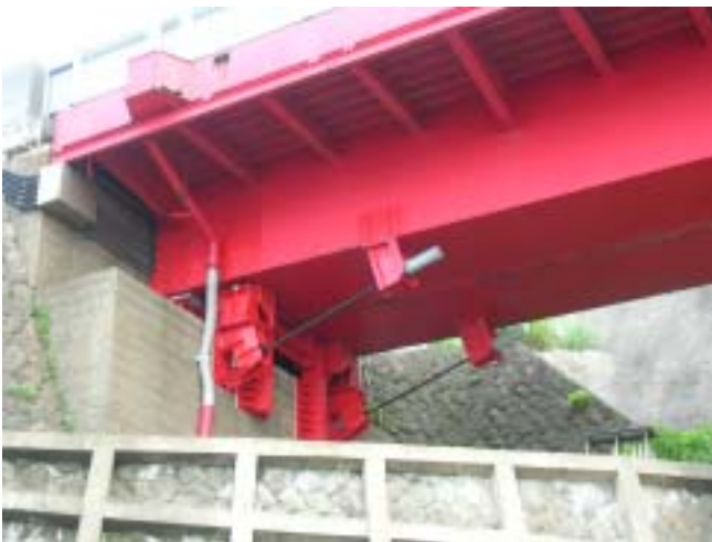
Photo 13 Unseating Prevention Devices (Cable Restrainers in Longitudinal and Uplift Directions)
