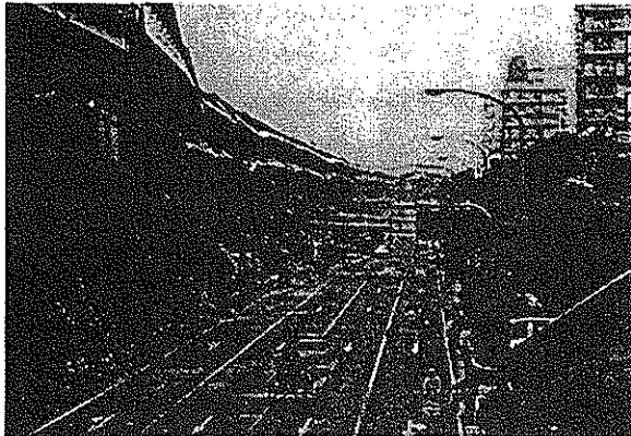
Photo. 5 Disruption of Arterial Viaduct
