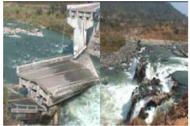
Figure 7. Spans Collapsed due to Fault Rupture
