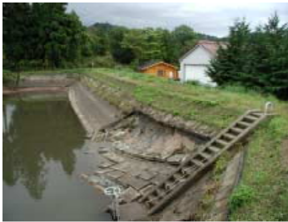
Photograph 12 Damage to the Kanayatani Dam
