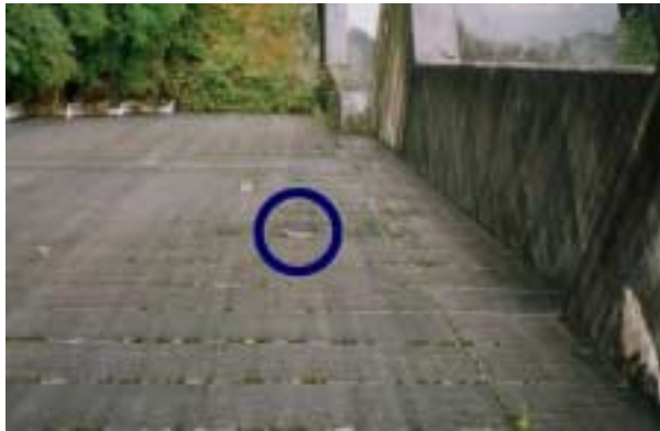
Photograph 7 Chipped Concrete on Downstream Surface of the Sugawara Dam
