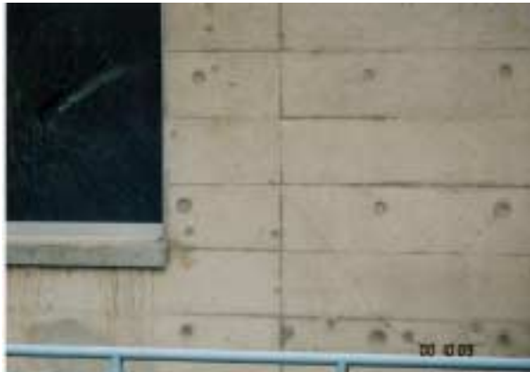
Photograph 3 An Example of Cracks on Wall of Guard Gate House of the Kasho Dam (exterior wall surface on the right bank side)
