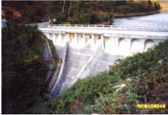
Photograph 9 Downstream View of the Uh Dam
