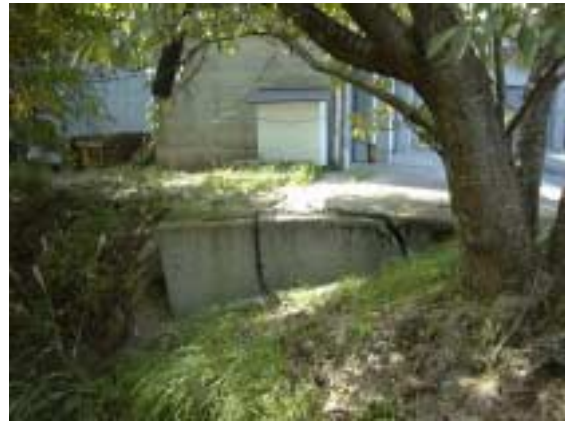
Photograph 8 An Example of Cracks in Ground Near the Sugawara Dam (near the garage on the downstream right bank)
