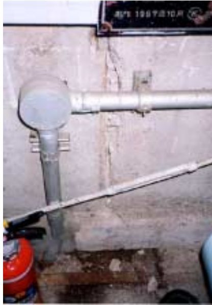
Photograph 6 Cracking on Wall of Guard Gate House of the Sugawara Dam (interior wall surface on the downstream side)
