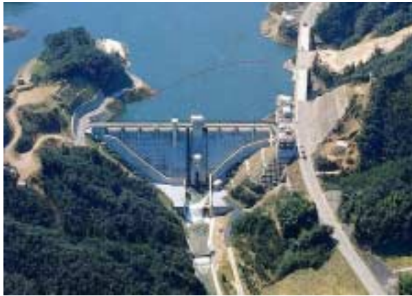
Photograph 1 View of the Kasho Dam
