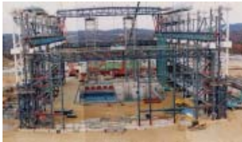
Fig. 2 Sliding Construction Method
