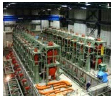
Fig. 6 Main Hydraulic Pump Units
