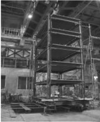
(a) Five-story test frame
