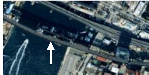
Fig-2 Shifted Girder at Kobe-Hamate Bypass (Simulated Image with 1m resolution)
