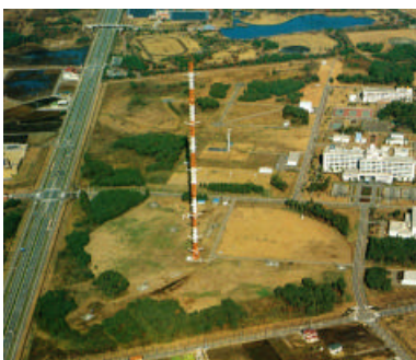
(b) Observation tower (MRI) with anemometers
