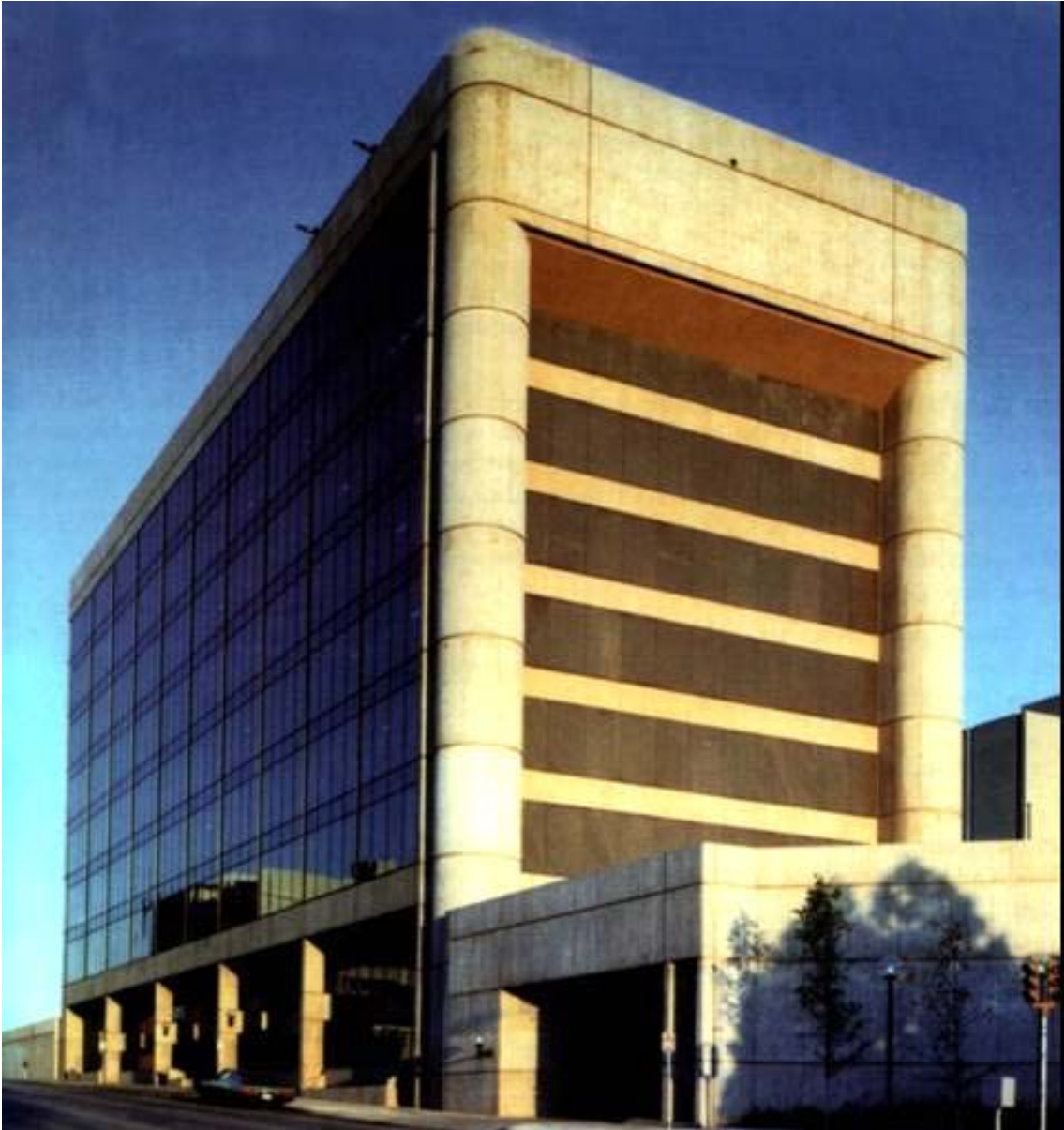
Figure 1. Murrah Building Prior to Blast.
