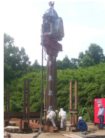
Fig.3 driving the pile with vibrohammer (Top piece of pile)
