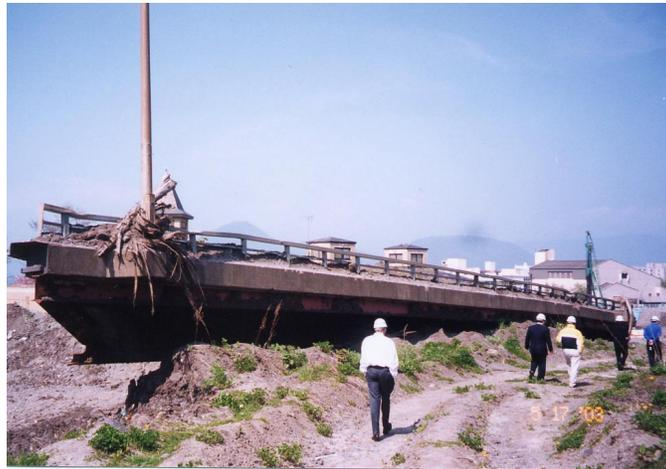
Figure 7. Bridge Washed Away by Mudflow.
