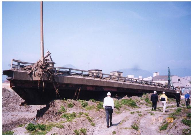
Figure 7. Bridge Washed Away by Mudflow.
