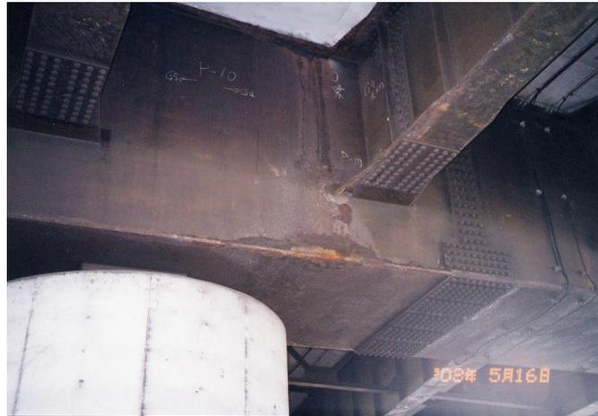
Figure 5. Viaduct Using Weather Resistant Steel.
