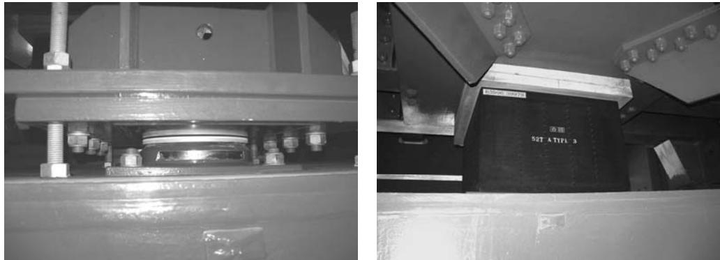
Photos of a newly installed sliding isolation bearing (left) and a rubber isolation bearing (right). Photo taken by M. Todorovska
