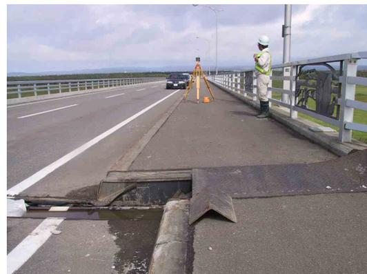
Photo 6 Damage of bearings and transverse residual displacement of deck (about 70cm) (Tokachi River Bridge)
