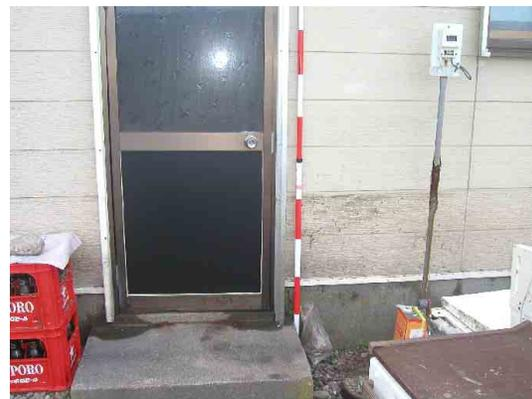
Photo 1 Evidence of tsunami run-up at Tokachi Port
