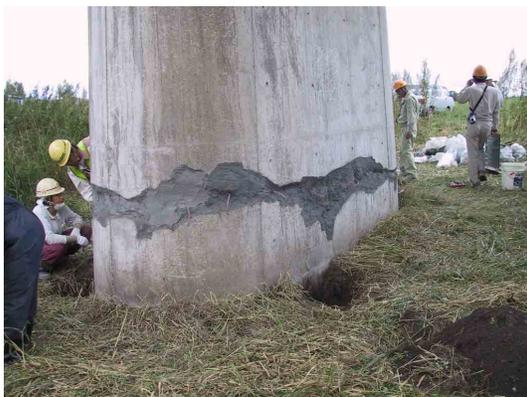
Photo 5 Damage of wall-type reinforced concrete columns (Chiyoda Bridge). Spall-off of cover concrete was repaired by concrete injection.)
