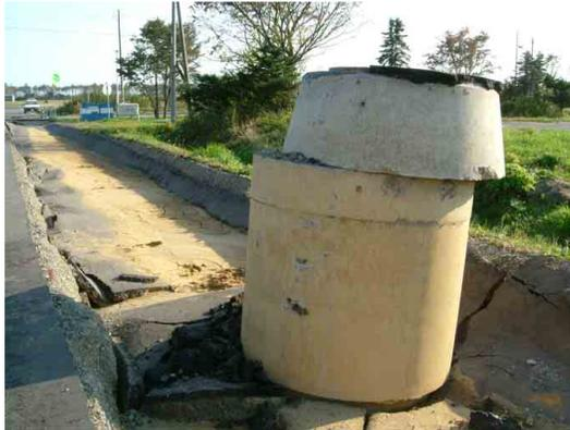
Photo 9 Ejected manhole and settlement of road surface
