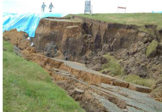
Photo 4 Collapse of slope of Tokachi river dike (right bank, 3.5 km from river mouth)
