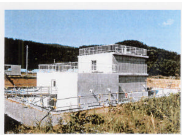
Fig.2 : A Typical Test example of SSI (Soil-Structure Interaction) model test. "Model Test on Dynamic Cross Interaction Effects of Adjacent Structures"
