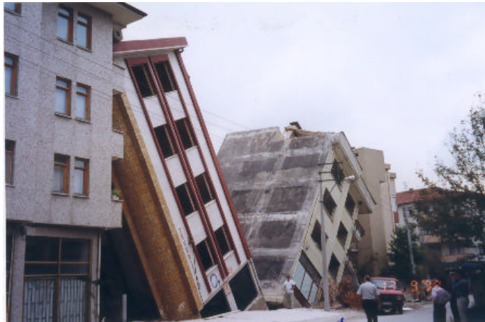
Figure 11. Settlement and overturning of buildings in Adapazari.
