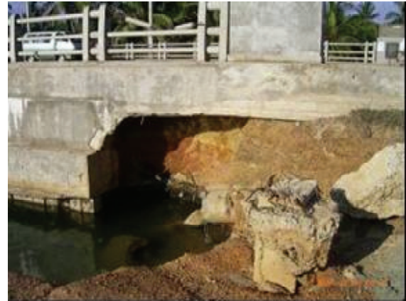
Photo-6. Scouring of a bridge (103Kp) (② in the map)
