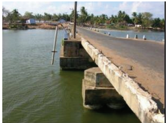
(1) The scoured out causeway mound (2) Damage to the sign post and curb Photo -2. The damage to the Koddaiikkallar Causeway
