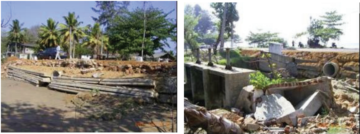
Photo -10. Damaged causeway with water pipes (145Kp ⑦ in the map)
