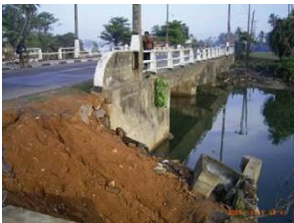
Photo-7. Erosion at approach (near 120Kp, ④ in the map)
