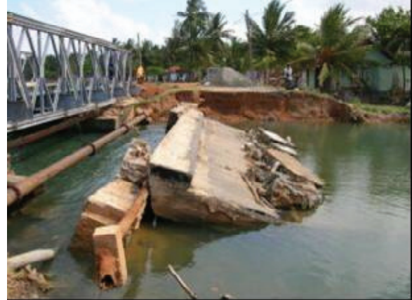
(1) Batticaloa Lagoon on the right. (2) The fallen bridge girder Photo-1. Collapsed simple digit bridge (Bar Road)
