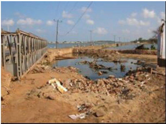
(1) The scoured out causeway mound (2) Damage to the sign post and curb Photo -2. The damage to the Koddaiikkallar Causeway
