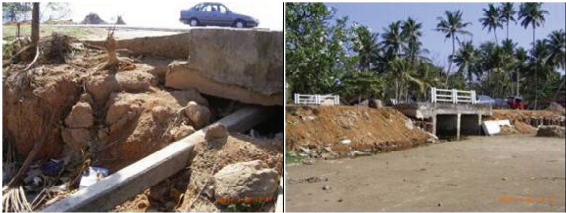
Photo-9. Culvert damaged (144Kp ⑥ in the map)
