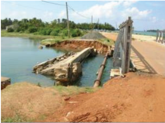
(1) Batticaloa Lagoon on the right. (2) The fallen bridge girder Photo-1. Collapsed simple digit bridge (Bar Road)
