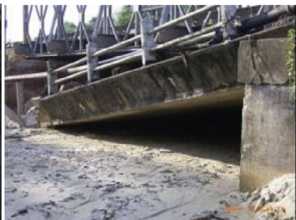
Photo-8. Bridge collapse due to erosion (137Kp ⑤ in the Map)
