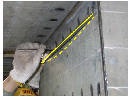
Fig.15 Local buckling at inner flange in C2 in column of C2 (+5 \delta_y )
