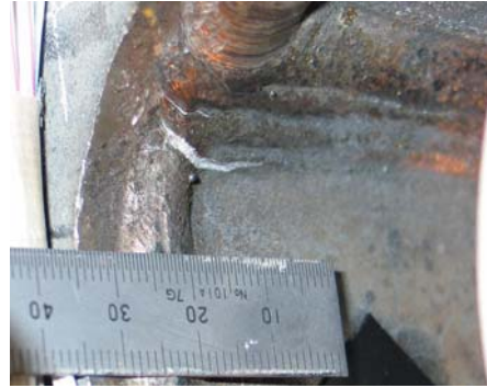
Fig.13 Cracks on flange side surface of weld bead in C2 (-3 \delta_y )
