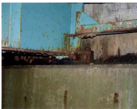
a. End of girder
