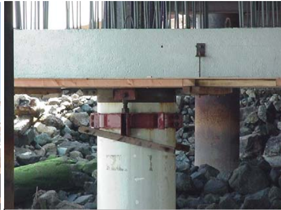
FIGURE 10 – PRE-CAST BENT CAP BEAM SUPPORTED ON SHAFT EXTENSIONS.
