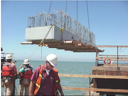
FIGURE 9 – PRE-CAST PORTION OF THE BENT CAP BEAM.
