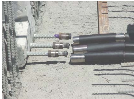
FIGURE 15 - MECHANICAL COUPLERS FOR MAIN GIRDER REINFORCEMENT.
