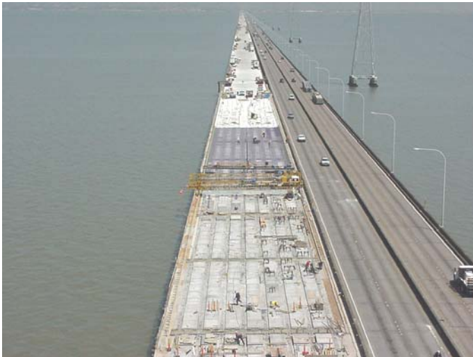
FIGURE 17 - SAN MATEO BRIDGE NEAR COMPLETION.
