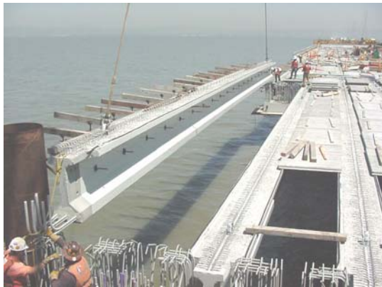
FIGURE 11 - PRE-CAST GIRDERS PLACED IN CAP BEAM OPENINGS.
