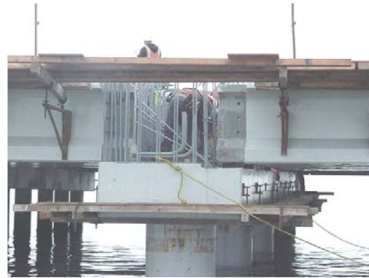
FIGURE 12 - ALL PRE-CAST ELEMENTS PLACED IN DESIGNATED OPENINGS.
