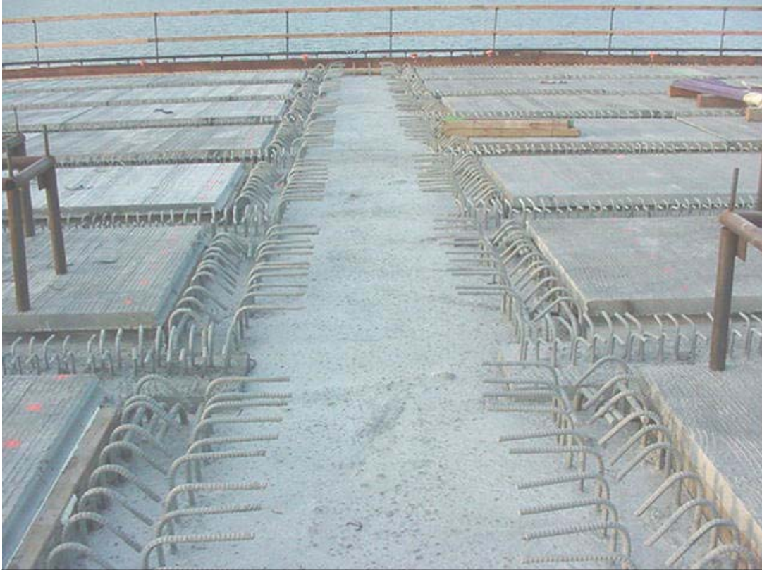
FIGURE 16 - VIEW OF COMPLETED BENT CAP BEAM READY FOR TOP REINFORCEMENT.
