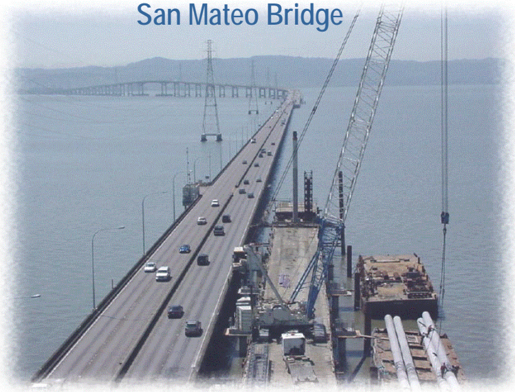
FIGURE 6 – SAN MATEO – HAYWARD BRIDGE.
