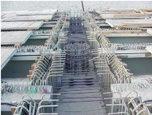
FIGURE 14 - CAST-IN-PLACE PORTION OF BENT CAP BEAM READY FOR CONCRETE POUR.
