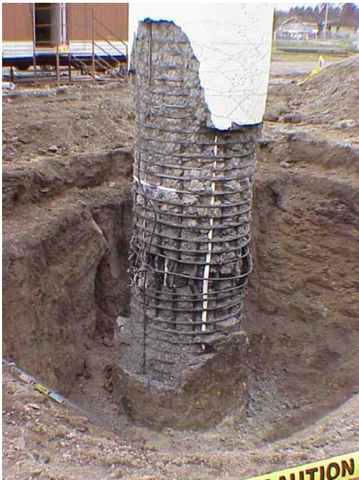
FIGURE 2 - PLASTIC HINGE BELOW GROUND.
