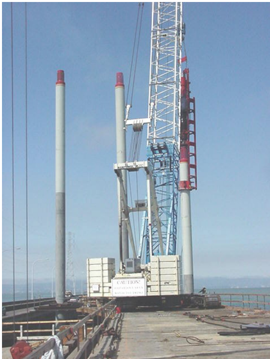
FIGURE 7 - 42-INCH HOLLOW SHELL COLUMN/SHAFT DRIVING OPERATION.
