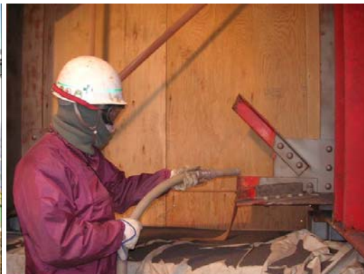
FIGURE 14. EXPERIMENT OF PARTIAL PAINTING AT EDGES OF GIRDERS (Adjustment of substrate)
