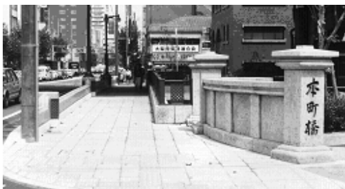
Figure 4. Bridge face of Honmachi Bridge
