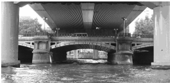
Figure 3. Side of Honmachi Bridge
