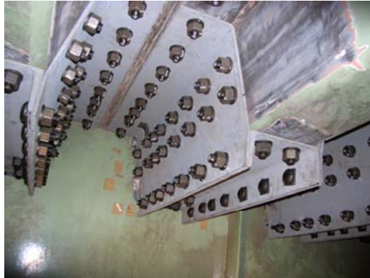
(b)Completed rib repair
