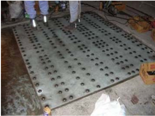
(a)Completed deck repair
