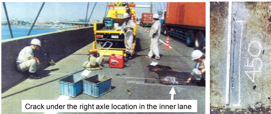
(a)After removing pavement
