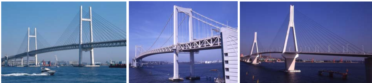
Yokohama Bay Bridge
