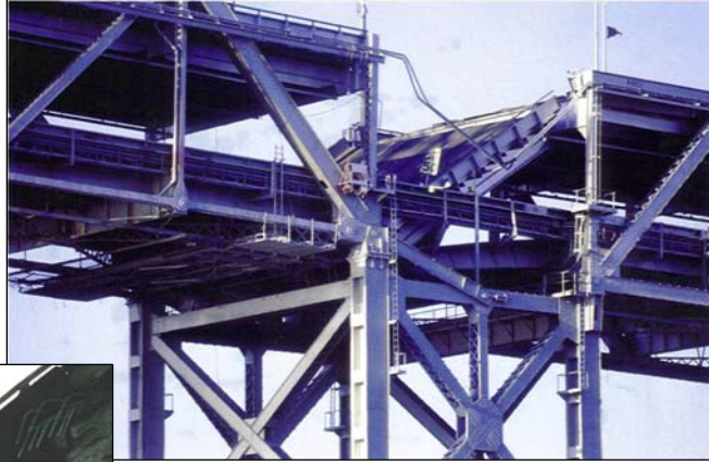
Figure 1 (right). Collapse of the link span at Tower E9 of the San Francisco Oakland Bay bridge due to inadequate seat lengths and anchor bolts.
