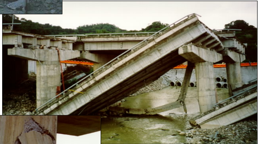
Figure 3 (right). Collapse of end spans in the Shi Wei bridge in Taichung, due to ground failure and nearby fault rupture.
