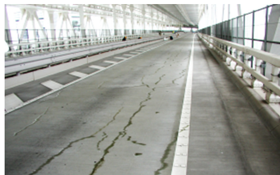
Photo 1 Acrylic-Injected SFRC Pavement on Yokohama Bay Bridge
