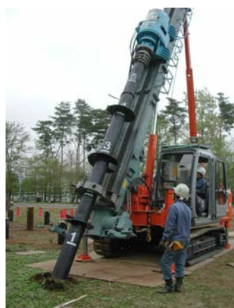
FIG. 1 MH-MP configuration PHOTO 1 Piling rig with MH-MP
