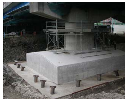
PHOTO 5 Pile cap extension
