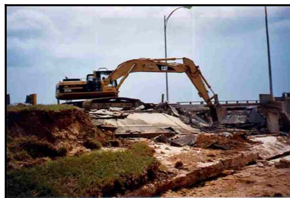
Figure 7 – Abutment and Approach Slab Repair
