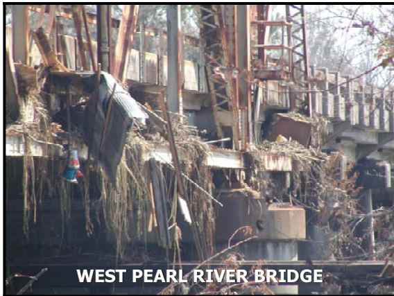
Figure 9 – Debris Buildup
