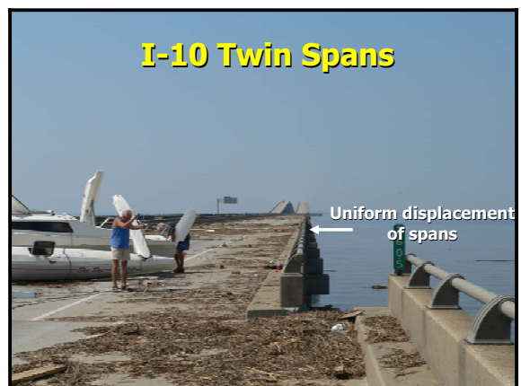
Figure 19 – Damage due to transverse wave action
