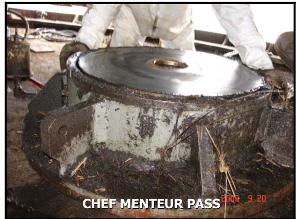
Figure 11 – Removal and Reconditioning of the Pivot Bearing
