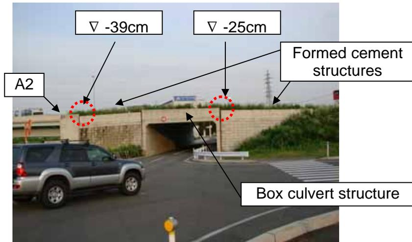
**Fig. 3** Box culvert structure nearby A2 abutment
