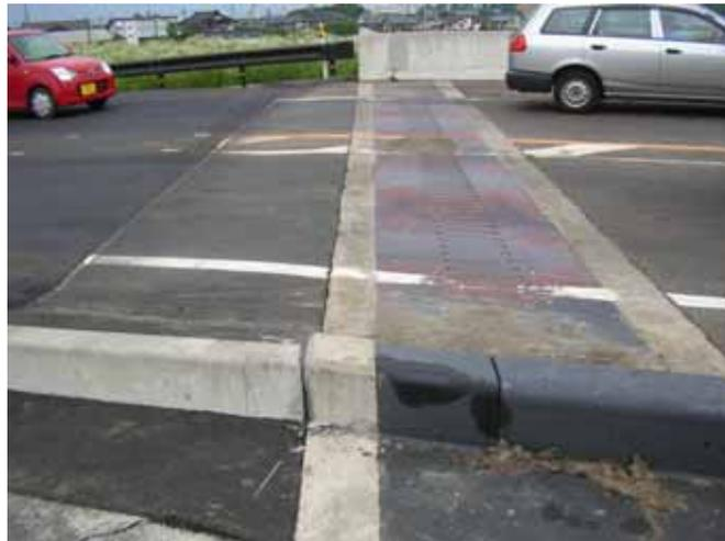
**Fig. 6 Clogging of expansion joint**
