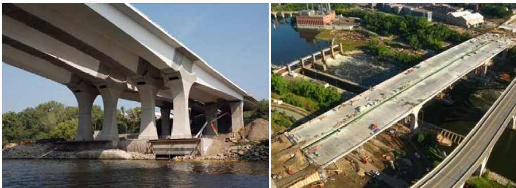
FIGURE 1: PHOTOS OF THE I35W ST. ANTHONY FALLS BRIDGE DURING CONSTRUCTION
