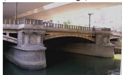
Photo 6 Honmachi Bridge (Oldest Bridge built in 1913)
