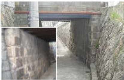
Photo3 E.g. of Masonry Abutment
