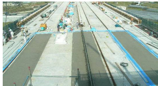
Photo-12 Cast-in-situ slab
