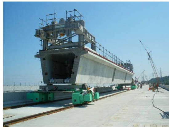
Photo-8 Transportation of the girder
