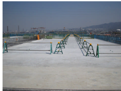
Photo-6 Cast-in-situ slab
