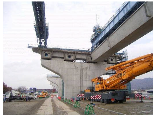
Photo-4 Transversal movement of the girder
