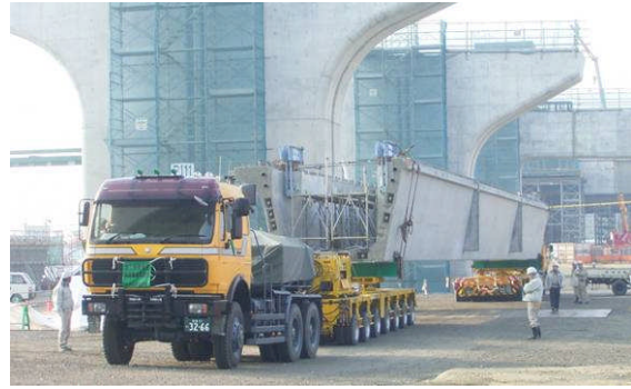
Photo-2 Transportation of the U-girder
