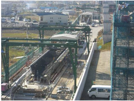
Photo-1 Casting yard
