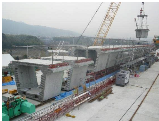
Photo-7 Assembling the segments
