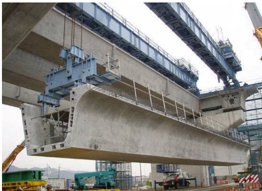
Photo-3 Erection of the U-girder
