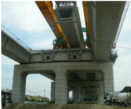
Photo-9 Erection of the girder
