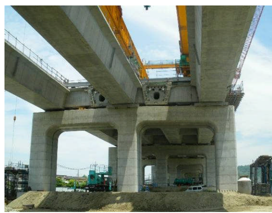
Photo-10 Transversal movement of the girder
