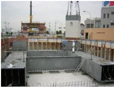
Steel Spread Foundation (Continuous Footing)
