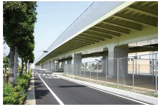
Full View of the Completed Viaduct
