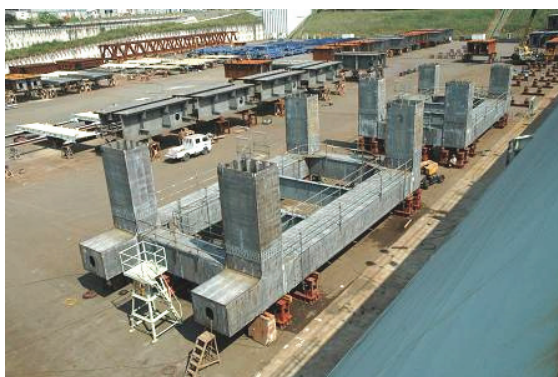
Fig. 5 Temporary Assembly for a Steel Spread Foundation (Harada Viaduct)
