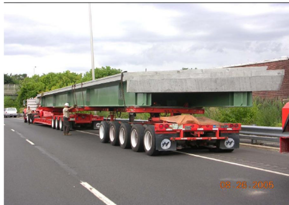
Figure 7 Prefabricated Modular Segment in Transportation
