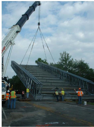
Figure 4 Temporary Bridge and Replacement Bridge Using Prefabricated system and Components
