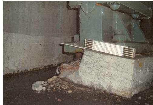
Figure 5 Deteriorated Decks of the Route 1 Bridge over the Olden Avenue Connector Figure 6 Deteriorated Pedestal of Bearings
