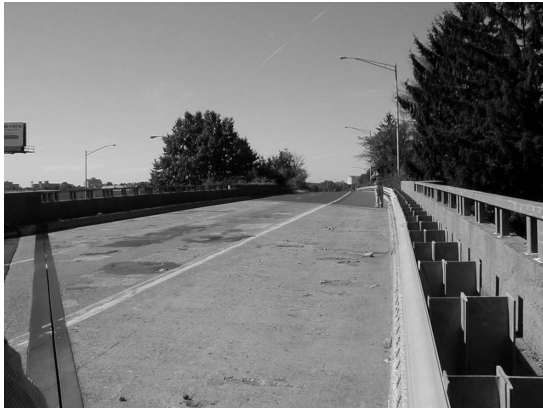
Figure 5 Deteriorated Decks of the Route 1 Bridge over the Olden Avenue Connector Figure 6 Deteriorated Pedestal of Bearings
