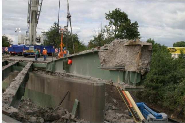
(a) Demolition/Removal of Existing Structure
