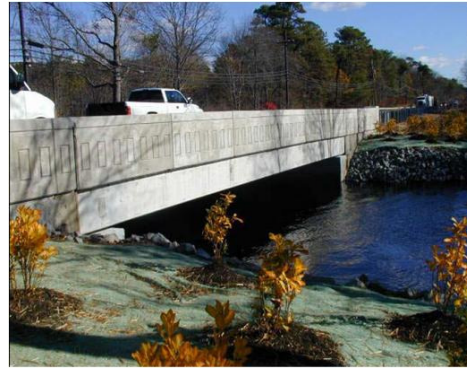
Figure 4 Temporary Bridge and Replacement Bridge Using Prefabricated system and Components
