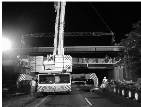
Figure 3 Night Time Erection of Modular Deck Panels Over I-295
