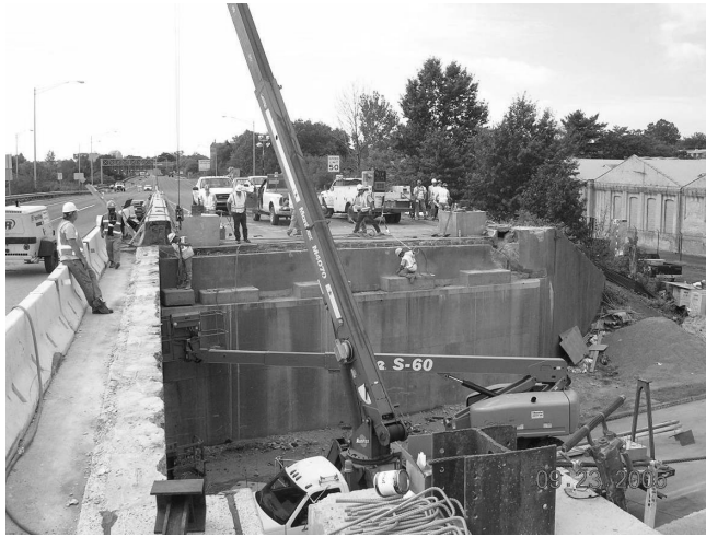
(b) Initiation of Erection of Route 1 Southbound Bridge over Mulberry Street
